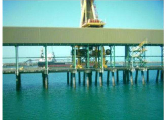
low water. Both berths are capable of handling vessels of 80, 000 tonnes. A suitable treatment was required to protect these valuable reinforced concrete structures from further chloride ion ingress caused by salt water spray and reducing costly maintenance work.
