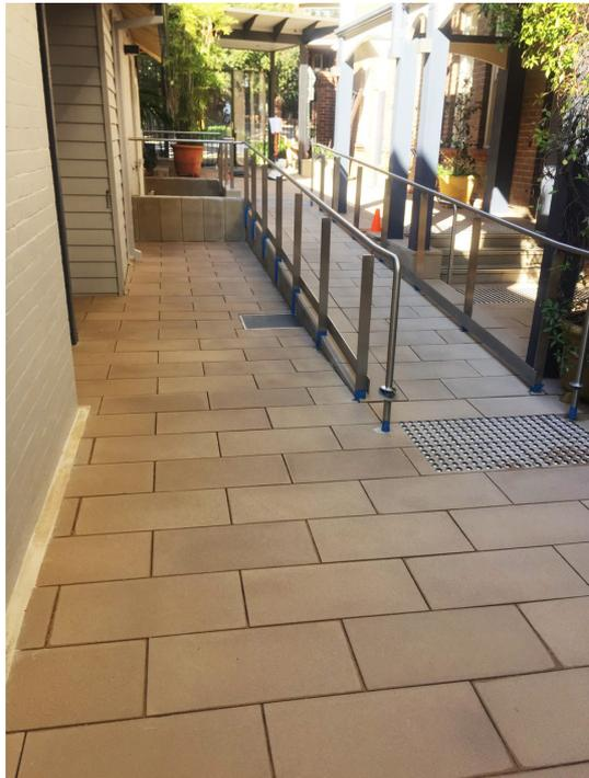
Simon and his team cleaned the new concrete pavers thoroughly and left it to dry. Once it was completely dry, the sealer was applied.
