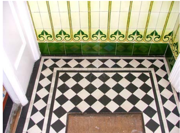
Victorian geometric encaustic tiles restoration Before-After
