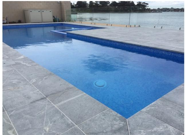
We normally do not recommend DRY-TREAT 40SK™ on granite as the consolidator will have trouble penetrating through denser materials. **A test should always be conducted on any and every sealing job in a small, conspicuous area.** In this instance, the test showed that the material was able to absorb DRY-TREAT 40SK.
