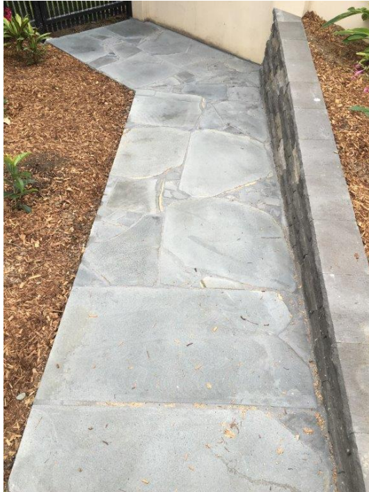
Walkway before grout haze cleaning and sealing
