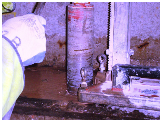
Fig. 5. Coring on top of a silane-treated RC cross-beam.
