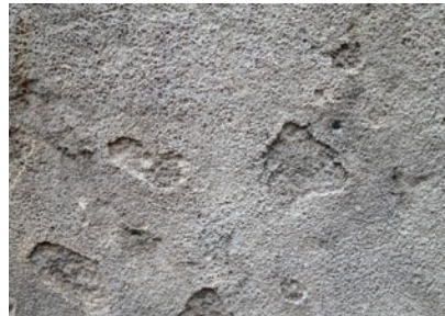
Freeze-thaw spalling
